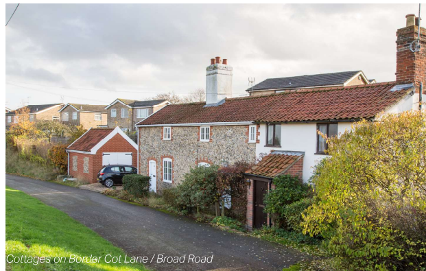
Cottages on Border Cot Lane / Broad Road
