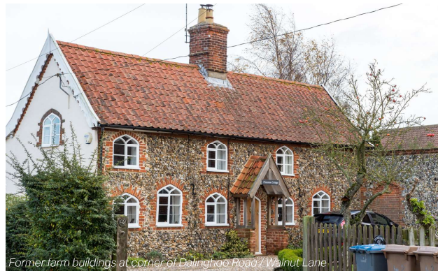
Former farm buildings at corner of Dallinghoo Road / Walnut Lane
